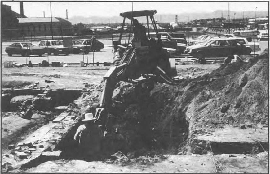
Figure 19 - Under the supervision of an archaeologist, a backhoe is used to carefully remove fill from a cellar.
