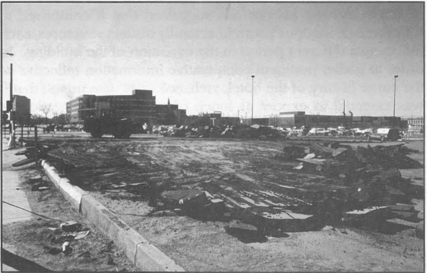
Figure 16 - Removing the asphalt parking surface that overlay the hotel site.
