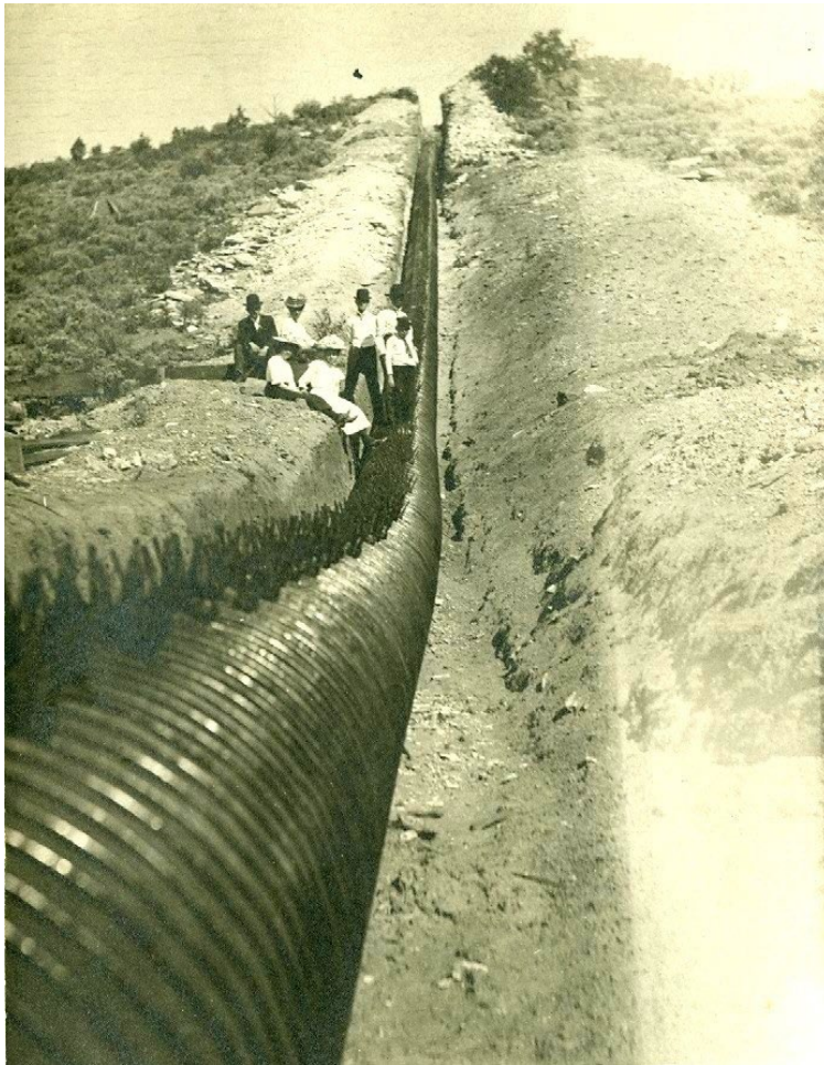
Figure 16. Wood stave pipe prior to burial.
