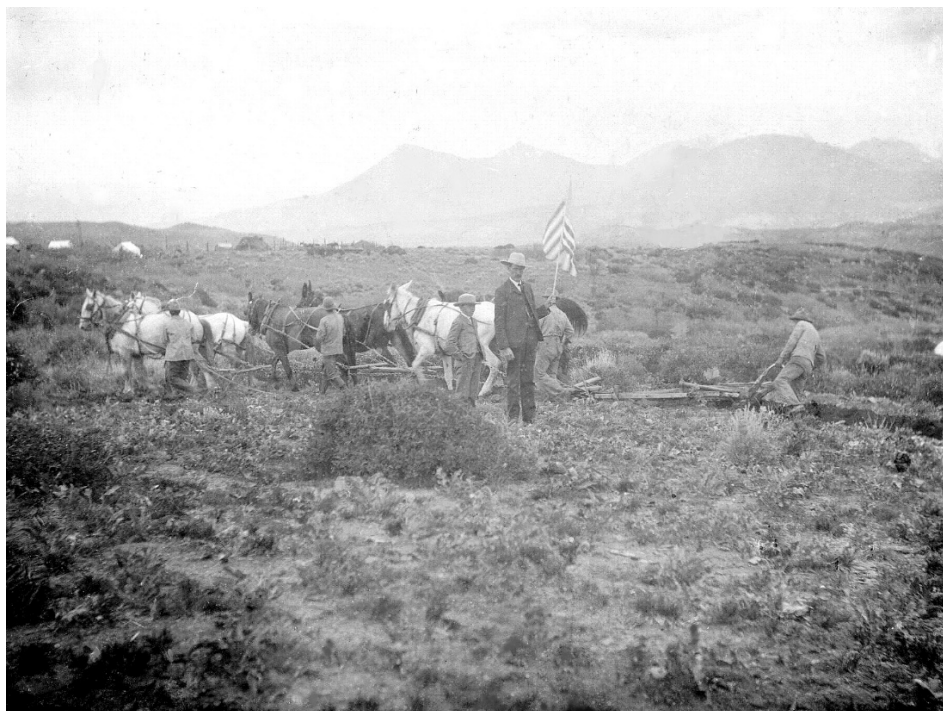
Figure 4. Excavation of open earthen canal, date unknown (early 1900s). Photo credit: Danny Cotten via Greg Powers, electronic version on file at ERO.
