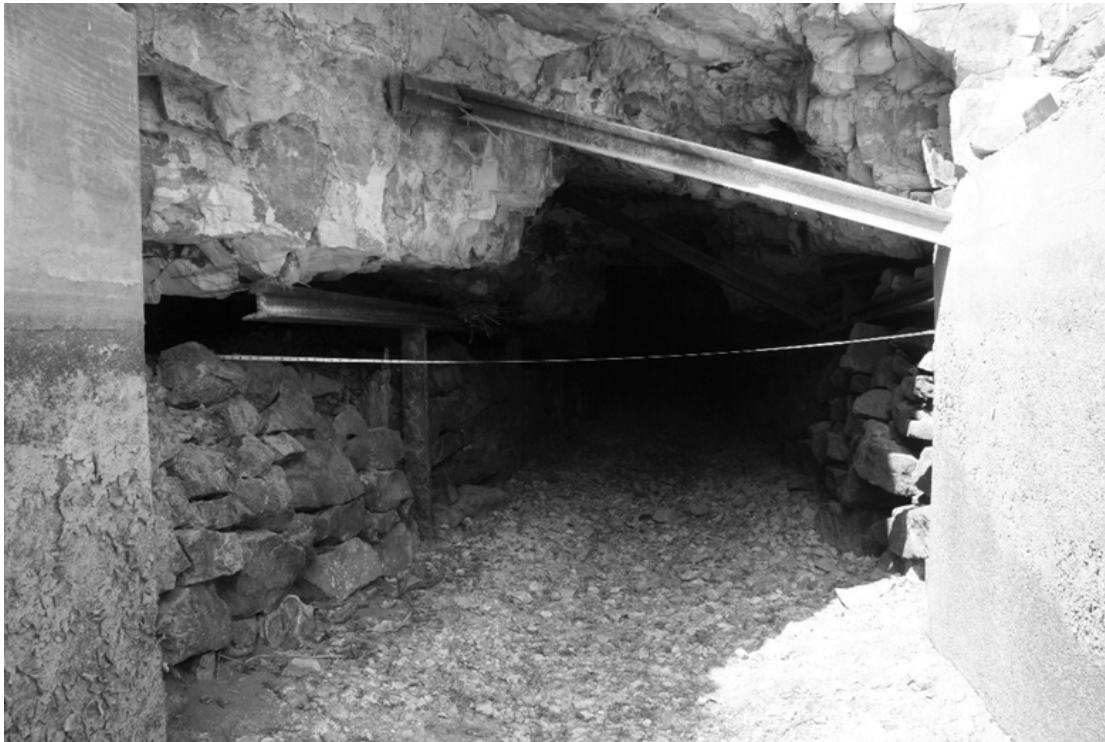
Figure 14. Profile of the canal at the upper tunnel opening, view to the north.
