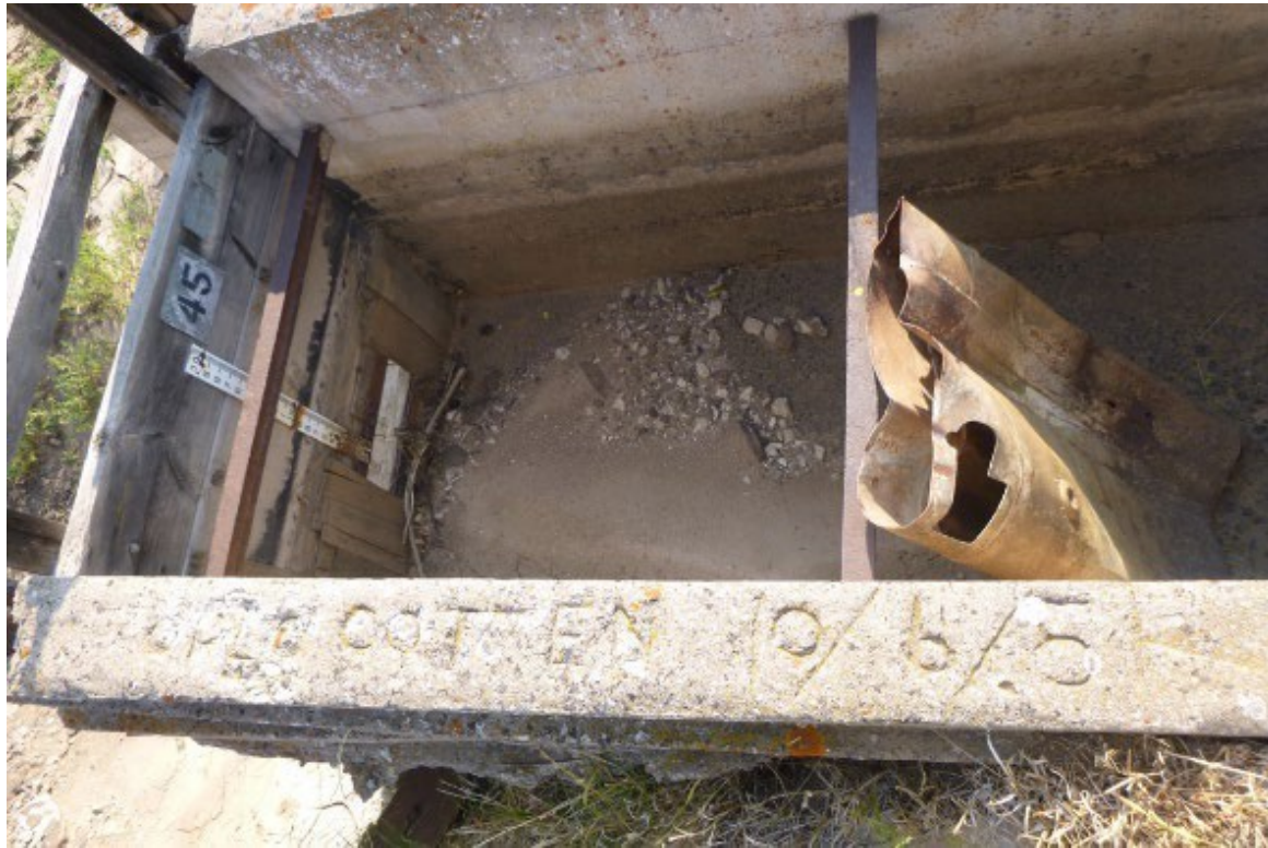
Figure 10. Headgate with “ORLO COTTEN” engraved in concrete.
