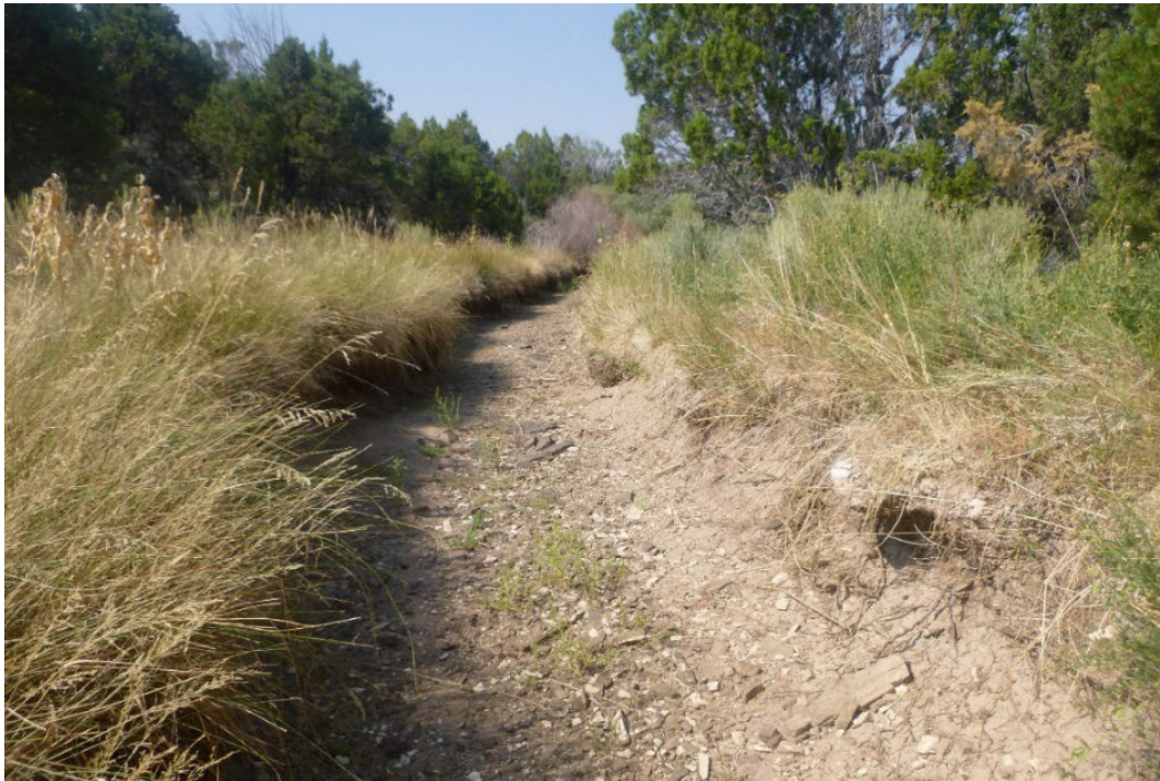
Figure 11. Gould Canal overview, view to the northeast.
