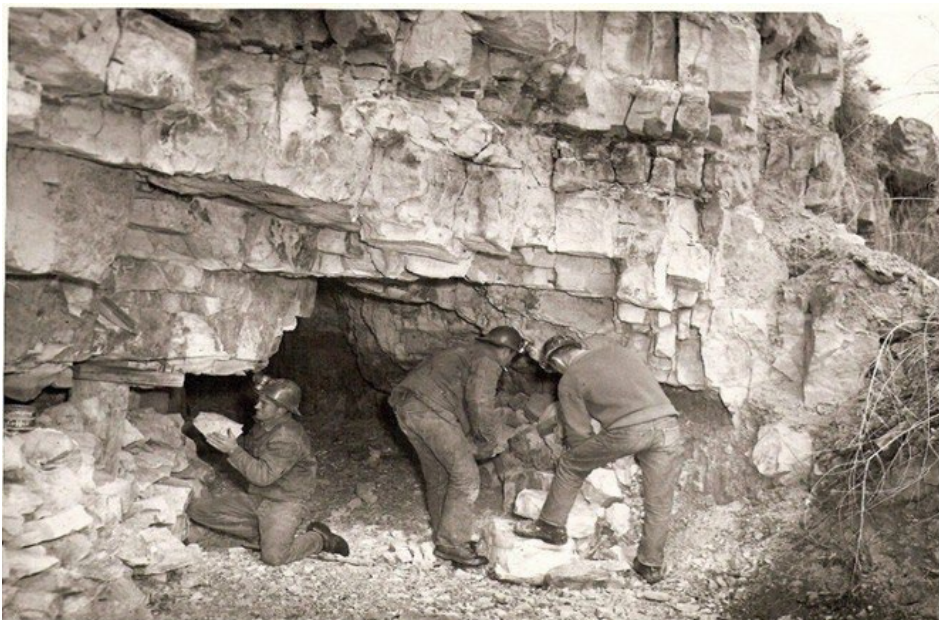
Figure 13. Tunnel construction or maintenance, date unknown (likely mid-1900s). Orlo “Babe” Cotten and Everett and George Howard are in the photo.
