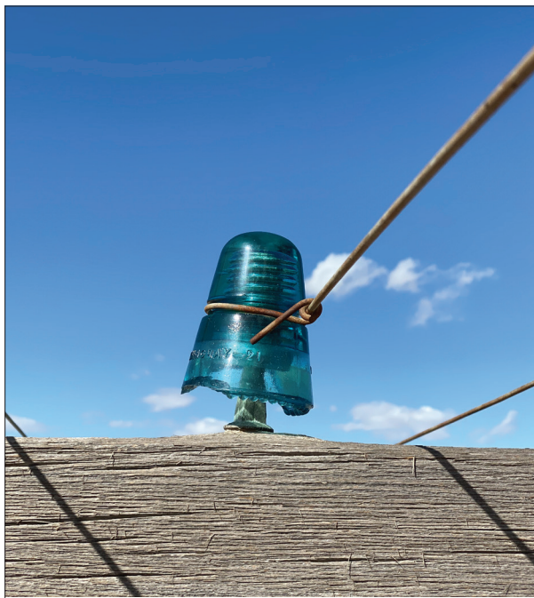
Figure 5. A strand of iron wire attached to a glass insulator on a communication line. (Photo by Joshua Birndorf.)
