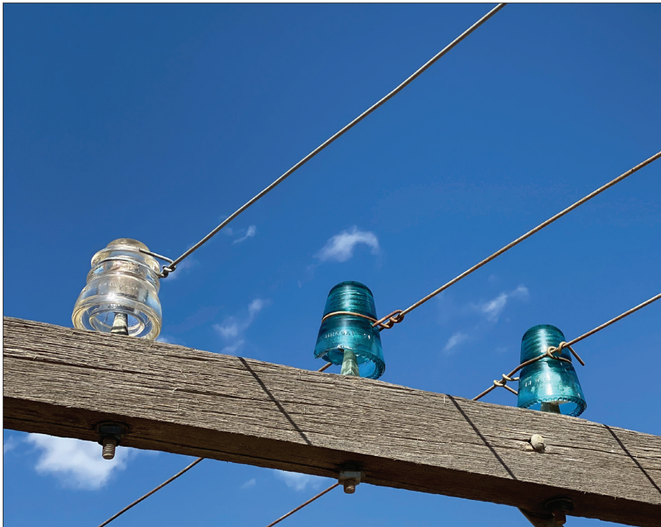
Figure 2. A communication line crossarm containing multiple insulators and iron wire. (Photo by Joshua Birndorf.)
