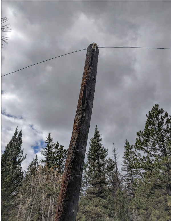
Figure 1. Communication pole associated with the Saguache-area site. Attached at the top of the pole are a glass insulator and iron wire. (Photo by Scott E. Ingram.)
