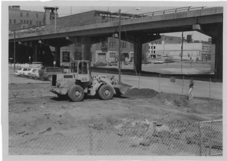
Figure 16 - Removal of asphalt blacktop prior to excavation; view to northeast.
