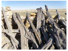
5LA.11853 Collapsed roof composed of unfinished timbers from native trees
