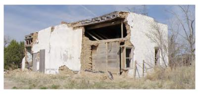
5LA.11913 Similar to the construction seen on homesteads, the Tyrone Store was constructed of adobe block covered in stucco
