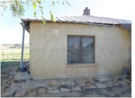
5OT.1104 House with corner cistern to collect runoff from the roof
