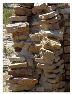
5LA.11676 Typical stone construction featuring a double laid wall
