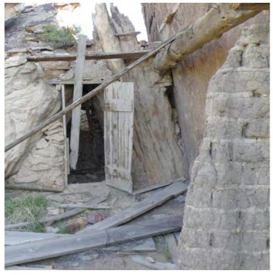
5LA.11673 View of structure incorporated into a rock overhang (Feature 1a) and adobe remnant wall represents addition
