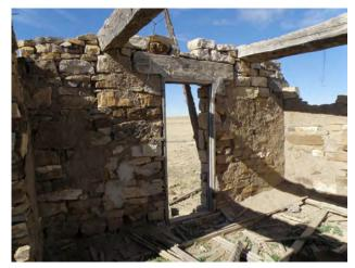
5LA.11857 Interior of a stone dwelling. Note remains of wood floor, interior adobe plaster, and large roof beams
