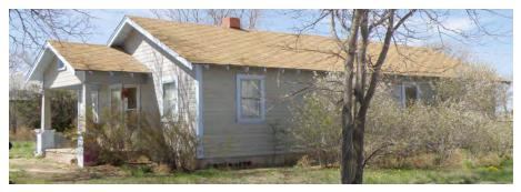
5LA.11920 Typical house in Kim. It is constructed of frame and features a small porch and exposed rafter tails.JPG
