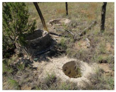
5LA.11759 Three associated concrete-lined cisterns on a pad, located west of Feature 1a. The larger cistern (center) has several Hutchinson stopper jar lids imbedded in the concrete base
