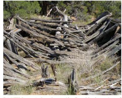
5LA.11759 Feature 1a, large dugout with collapsed Ponderosa pine roof main beam and juniper log roof joists
