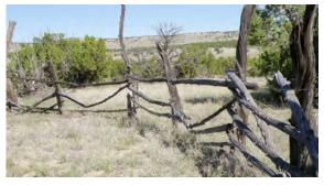
5LA.11715 Corral constructed of horizontal branches tied to tall wood posts with wire
