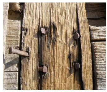
5HF.2336 Cut nail located on the depot's east wall confirming the structure's 19th century origin
