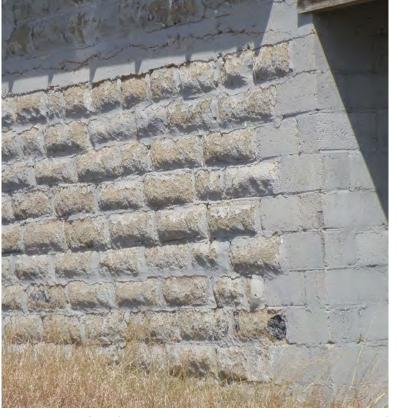
5LA.11923 This false front commercial building in Kim is constructed of concrete blocks. Many are rusticated giving them an appearance similar of that to the sandstone so common in the region
