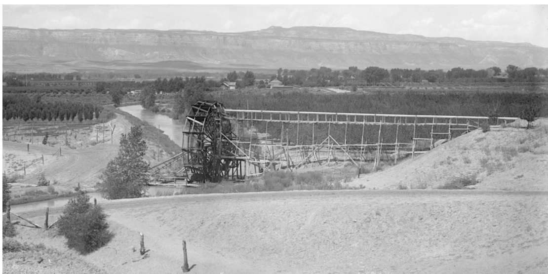
Figure 21. John Wellington's Wheel, constructed in 1894 to lift water from the Grand Valley Canal to his orchard above. Photographed c. 1907 by Louis Charles McClure.
