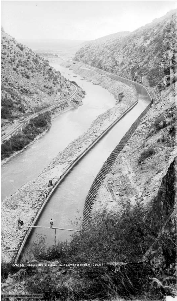
Figure 5. High Line Canal in Platte Canyon, circa 1883. Photographer: William Henry Jackson. A wooden bench flume carries the canal on a shelf blasted into the side of the canyon.
