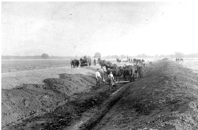
Figure 14. Ditch construction by teams of horses with fresno scrapers. Photographed 1918.
