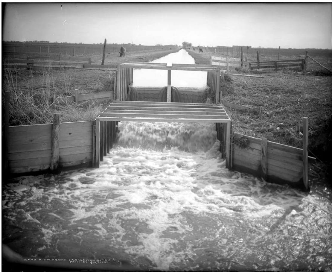
Figure 22. Simple wooden drop structure on a ditch on the eastern plains. Photographed c. 1900-1920 by Louis Charles McClure.
