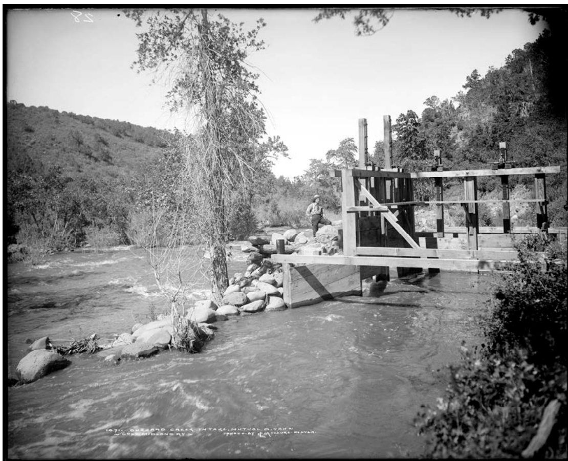
Figure 13. Headgate for Mutual Ditch on Buzzard Creek in Plateau Valley, Mesa County. Photographed by Louis Charles McClure c. 1911. Headgate is wooden with steel control mechanisms. Diversion works consist of a temporary rubble dam in the stream.
