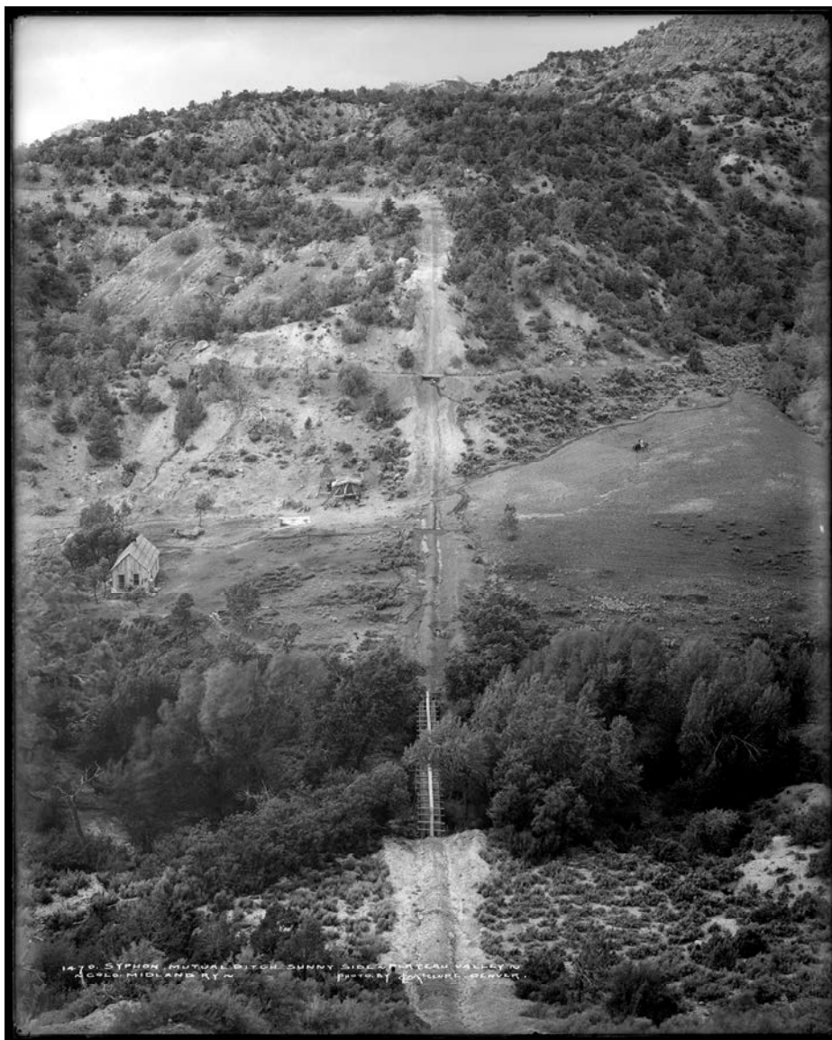
Figure 20. Mutual Ditch siphon, Sunnyside, in Plateau Valley, Mesa County. Photographed by Louis Charles McClure, c. 1911. A lower ditch crosses the siphon on a wooden flume, feeding a lateral that crosses the siphon again, on an earthen berm.
