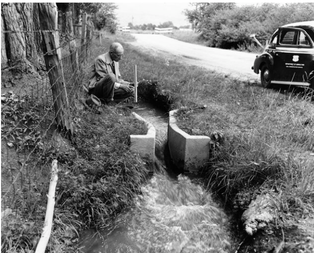
Figure 30. Professor Ralph Parshall with a concrete Parshall measuring flume, 1946.
