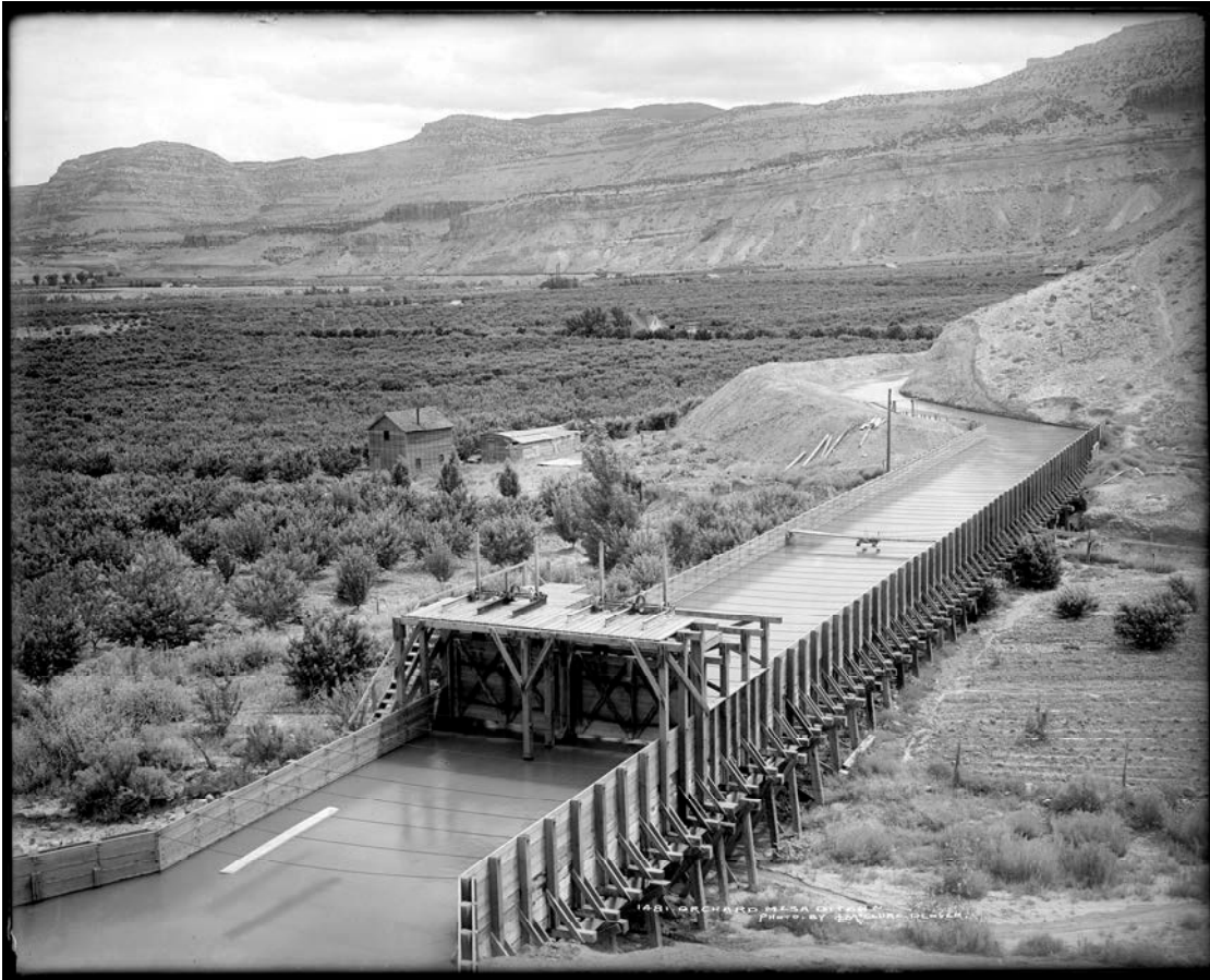
Figure 18. Large wooden flume on Orchard Mesa Canal, Mesa County. Photographed by Louis Charles McClure, c. 1911. The flume crosses a natural drainage and protects the canal from washing out.
