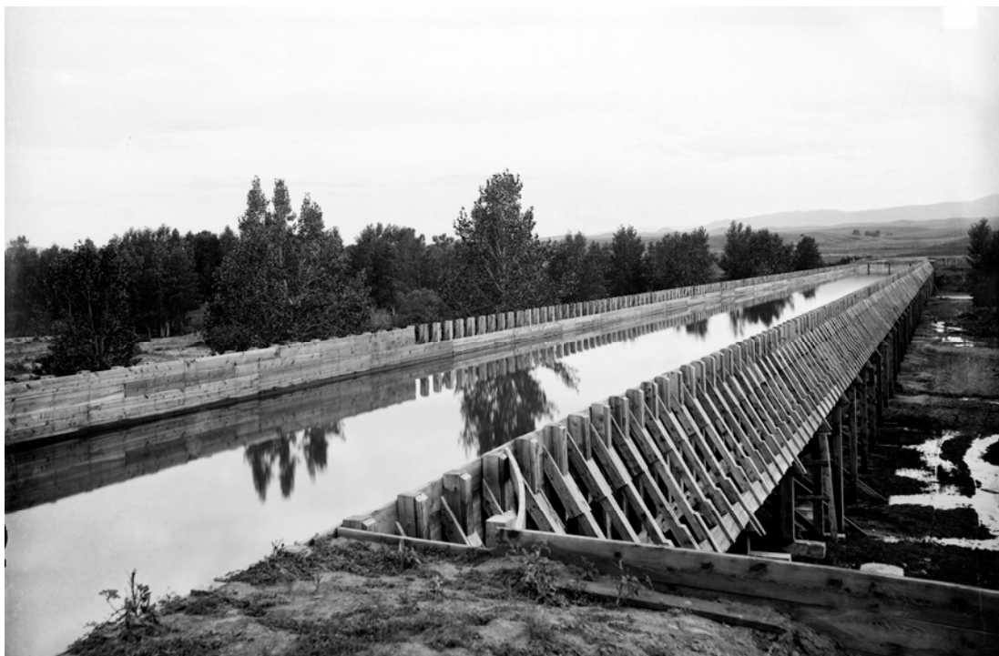
Figure 4. High Line Canal flume in Platte Canyon, Douglas County. Photographer: William Henry Jackson.
