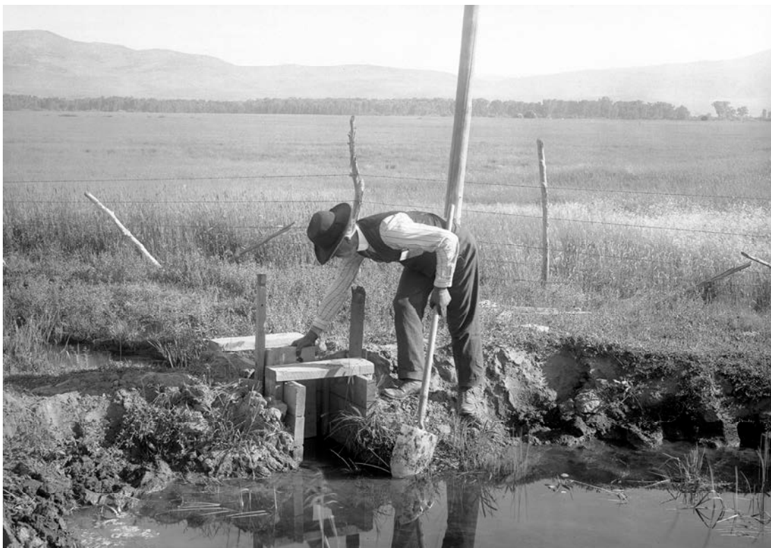
Figure 24. The simplest turnout: a small plank moved by hand in a wooden track. "Irrigation in Routt County," photographed by Louis Charles McClure, c. 1908-1915.
