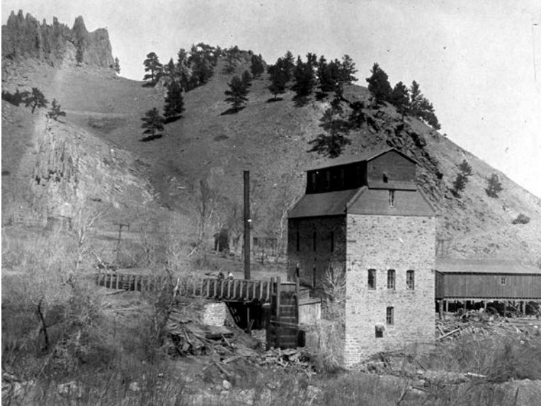
Figure 10. Yount Mill, Boulder, Photographed in 1900. The mill is powered by water from Farmers Ditch passing through a wooden flume and falling back into Boulder Creek.
