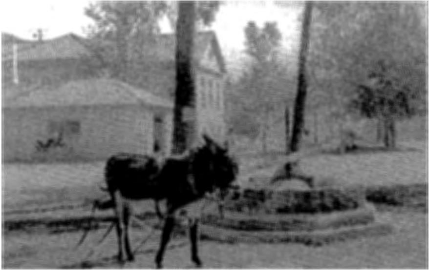
FIGURE 7. Relocated arrastra reported from the Dumont area (courtesy of the Denver Public Library, Western History Collection, Call Number X-60013).
